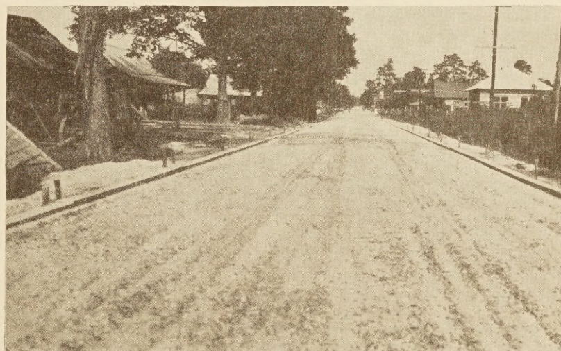
FIGURE 2.—PREPARATION FOR MIXED-IN-PLACE CONSTRUCTION ON SAND-CLAY BASE
